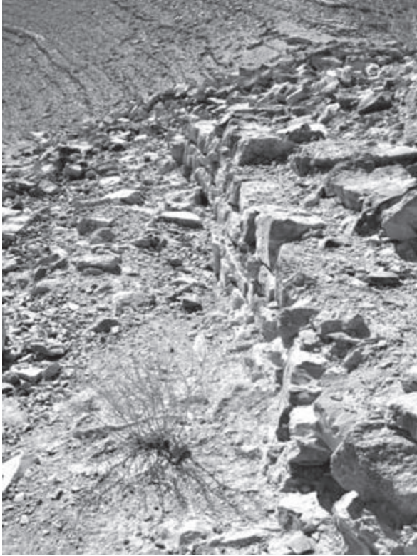
Figure 4.4. Fortification walls of al-Mu‘arradja.
